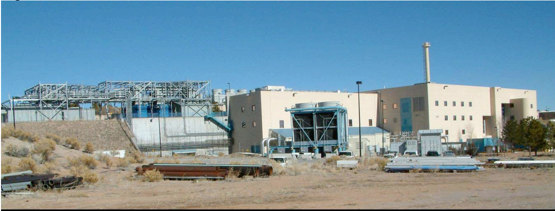
Figure 1 LEDA building at Los Alamos from the back showing the high bay areas, offices, and other facilities.
